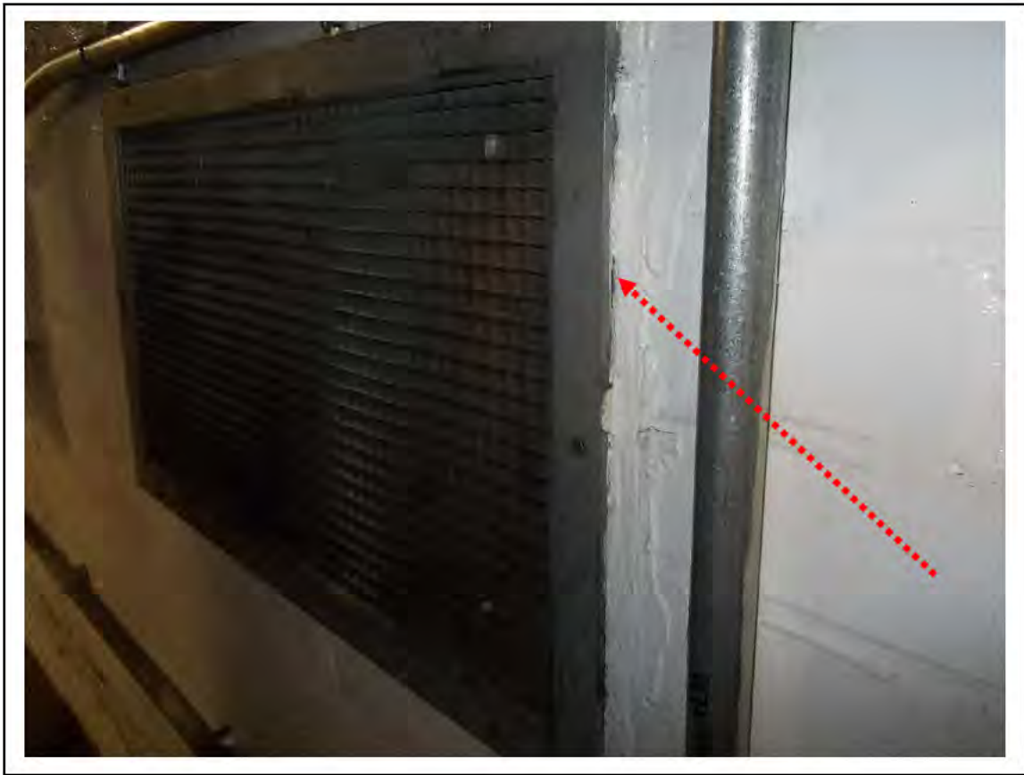
FIGURE 2: CONFIRMED ASBESTOS IN MASTIC IN UMC 1 & 2, 2/151 - DESCRIPTION & RESULT OF ASSESSMENT (SAMPLE REF. 110696/011111/02)
