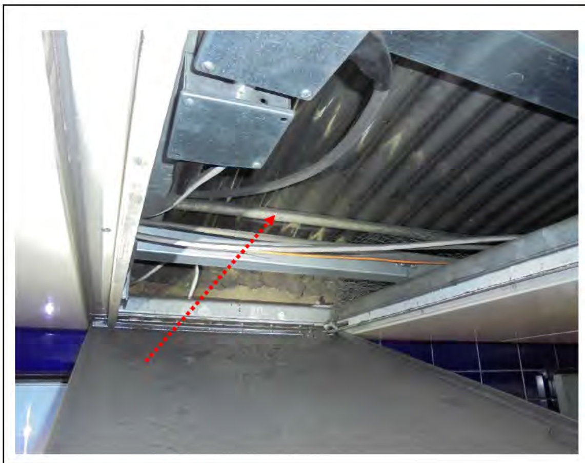
FIGURE 78: STRONGLY PRESUMED ASBESTOS IN CELLACTITE IN CIRC AREA AND PASSAGES, 6/081, 6/202 - 6/207 - DESCRIPTION & RESULT OF ASSESSMENT (SAMPLE REF. SP1 (10))
