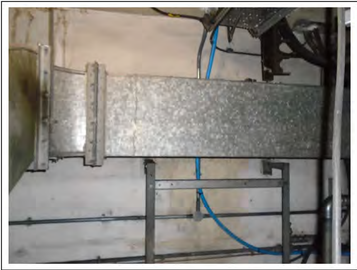
FIGURE 13: CONFIRMED ASBESTOS IN GASKETS IN UMC 3, 4, 5, 4/161 - DESCRIPTION & RESULT OF ASSESSMENT (SAMPLE REF. 100558/121010/14)
