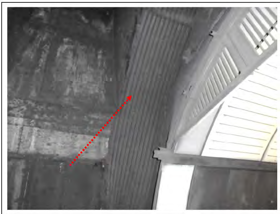
FIGURE 75: KNOWN ASBESTOS IN CELLACTITE IN PLATFORM 4, 6/262 - DESCRIPTION & RESULT OF ASSESSMENT (SAMPLE REF. K1 (10))
