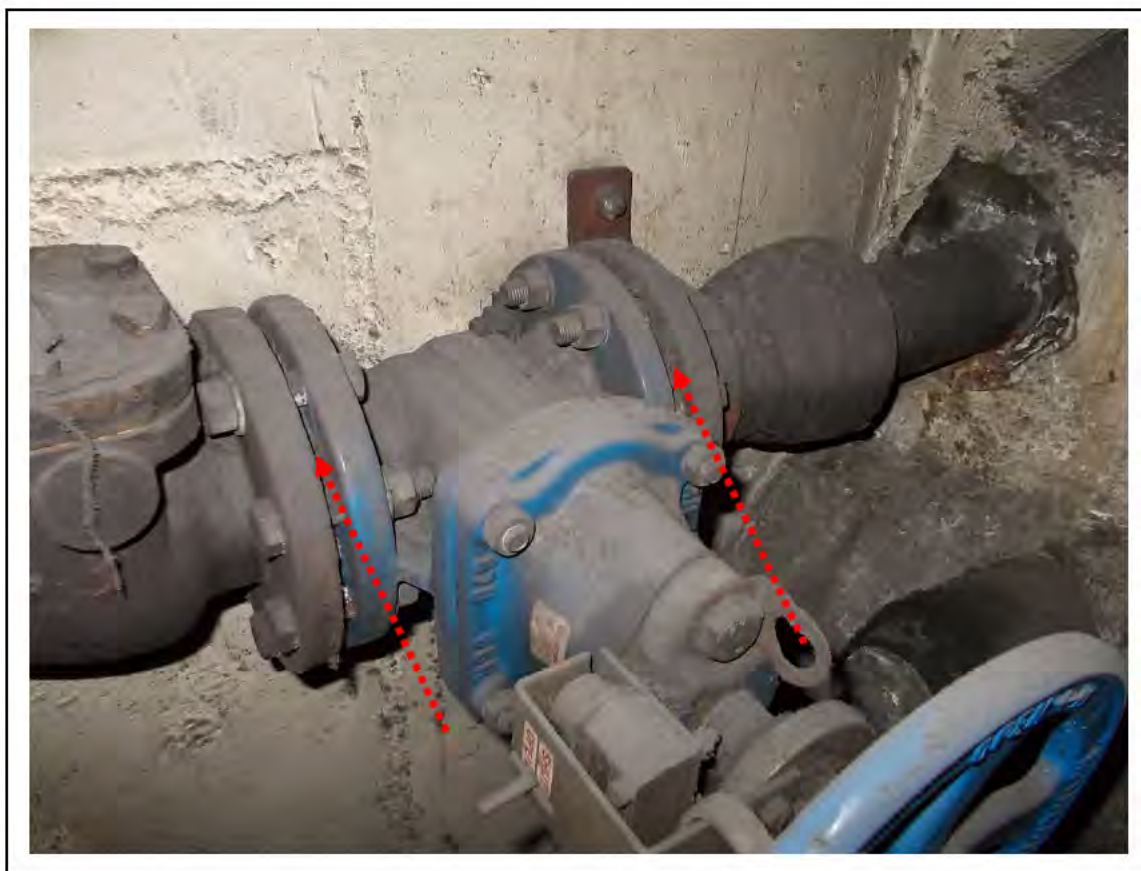
FIGURE 6: CONFIRMED ASBESTOS IN GASKETS IN UMC 6, 7, 8, 2/152 - DESCRIPTION & RESULT OF ASSESSMENT (SAMPLE REF. 161057/280616/02)
