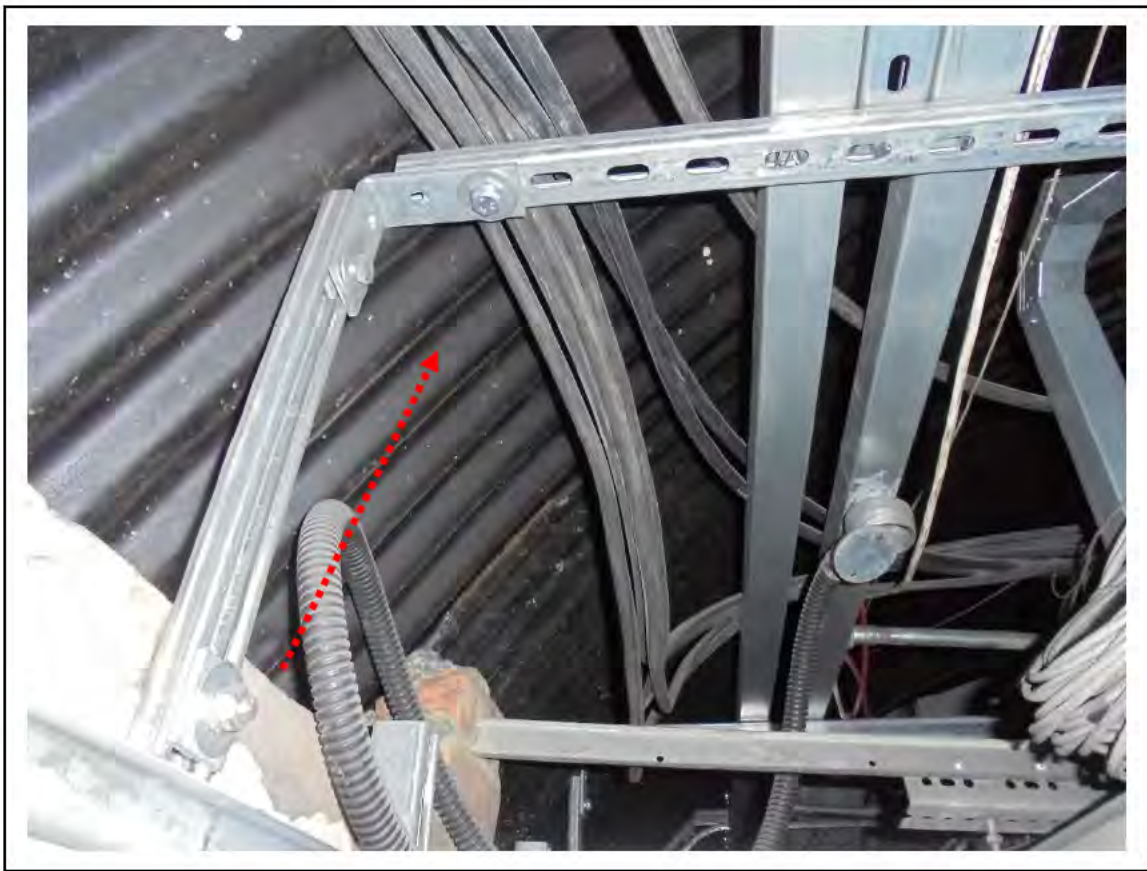
FIGURE 50: KNOWN ASBESTOS IN CELLACTITE SHEETING IN PASSAGE, 6/236 - DESCRIPTION & RESULT OF ASSESSMENT (SAMPLE REF. K1 (6))
