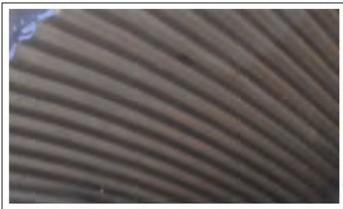
FIGURE 3: CONFIRMED ASBESTOS IN CELLACTITE IN UMC 1 & 2, 2/151 - DESCRIPTION & RESULT OF ASSESSMENT (SAMPLE REF. 110597/011011/01)
