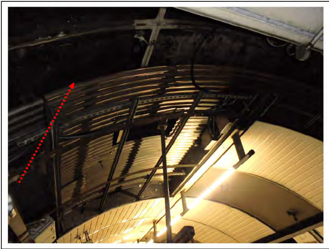
FIGURE 73: CONFIRMED ASBESTOS IN CELLACTITE IN PLATFORM 3, 6/261 - DESCRIPTION & RESULT OF ASSESSMENT (SAMPLE REF. ECS 85287 & 100946/210311/01)
