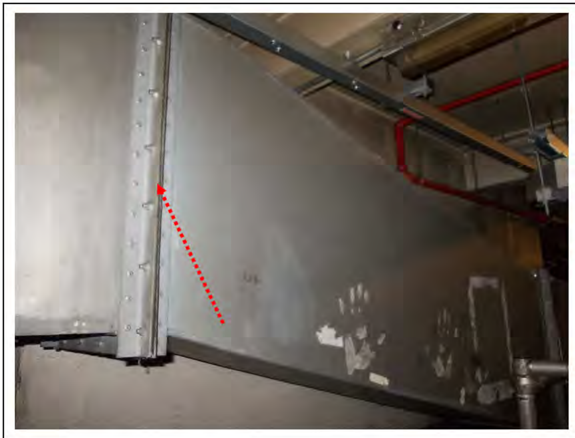
FIGURE 7: CONFIRMED ASBESTOS IN MASTIC IN UMC 6, 7, 8, 2/152 - DESCRIPTION & RESULT OF ASSESSMENT (SAMPLE REF. 100675/251110/06)
