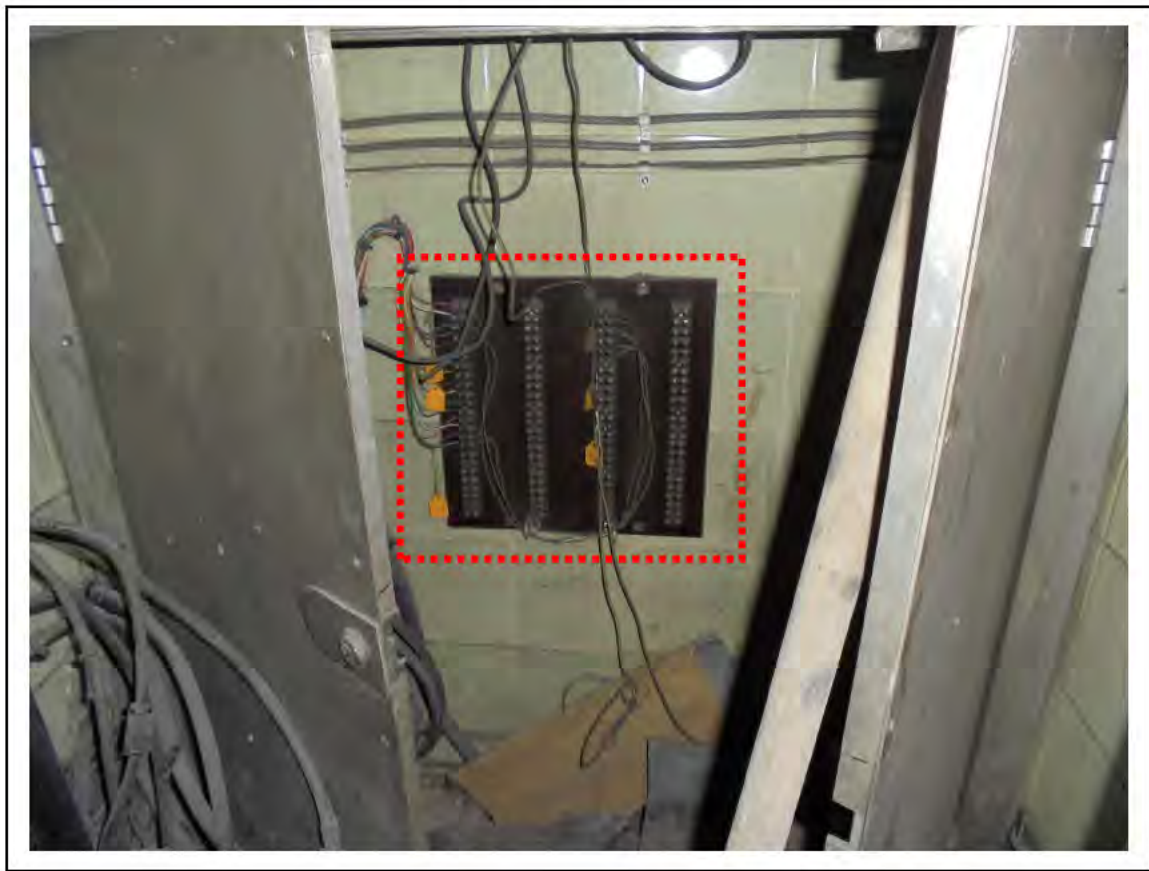
FIGURE 51: CONFIRMED ASBESTOS IN OLD BROWN COMPOSITE BOARD IN PASSAGE, 6/236 - DESCRIPTION & RESULT OF ASSESSMENT (SAMPLE REF. 161057/191116/01)
