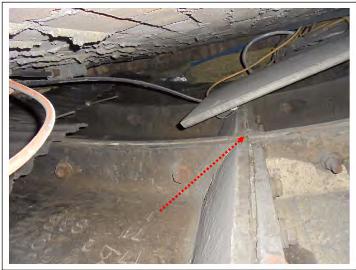
FIGURE 84: CONFIRMED ASBESTOS IN CAULKING IN BOSTWICK GATE CHAMBER, 4/765 - DESCRIPTION & RESULT OF ASSESSMENT (SAMPLE REF. SP1 & 2 (2))
