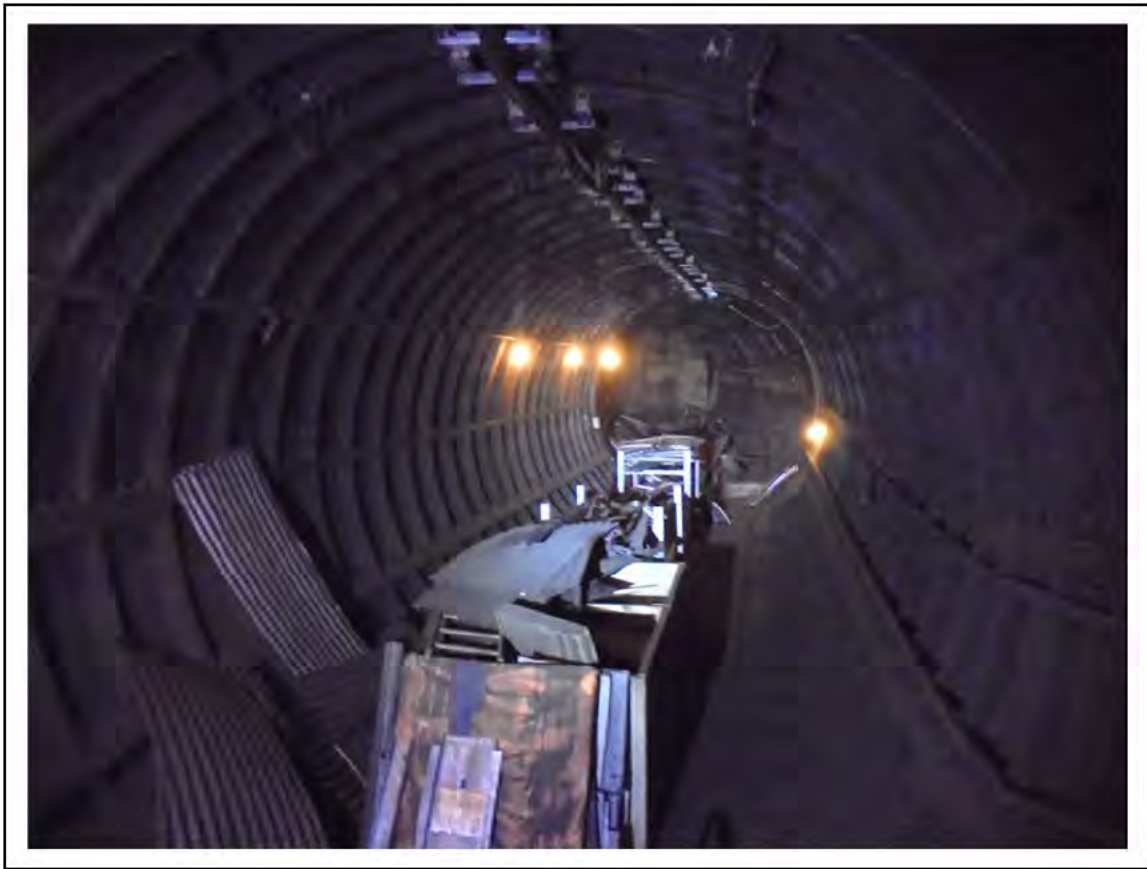
FIGURE 49: CONFIRMED ASBESTOS IN CAULKING TO TUNNEL RINGS IN DRAFT RELIEF TUNNEL, 4/793 - DESCRIPTION & RESULT OF ASSESSMENT (SAMPLE REF. 051008/7)
