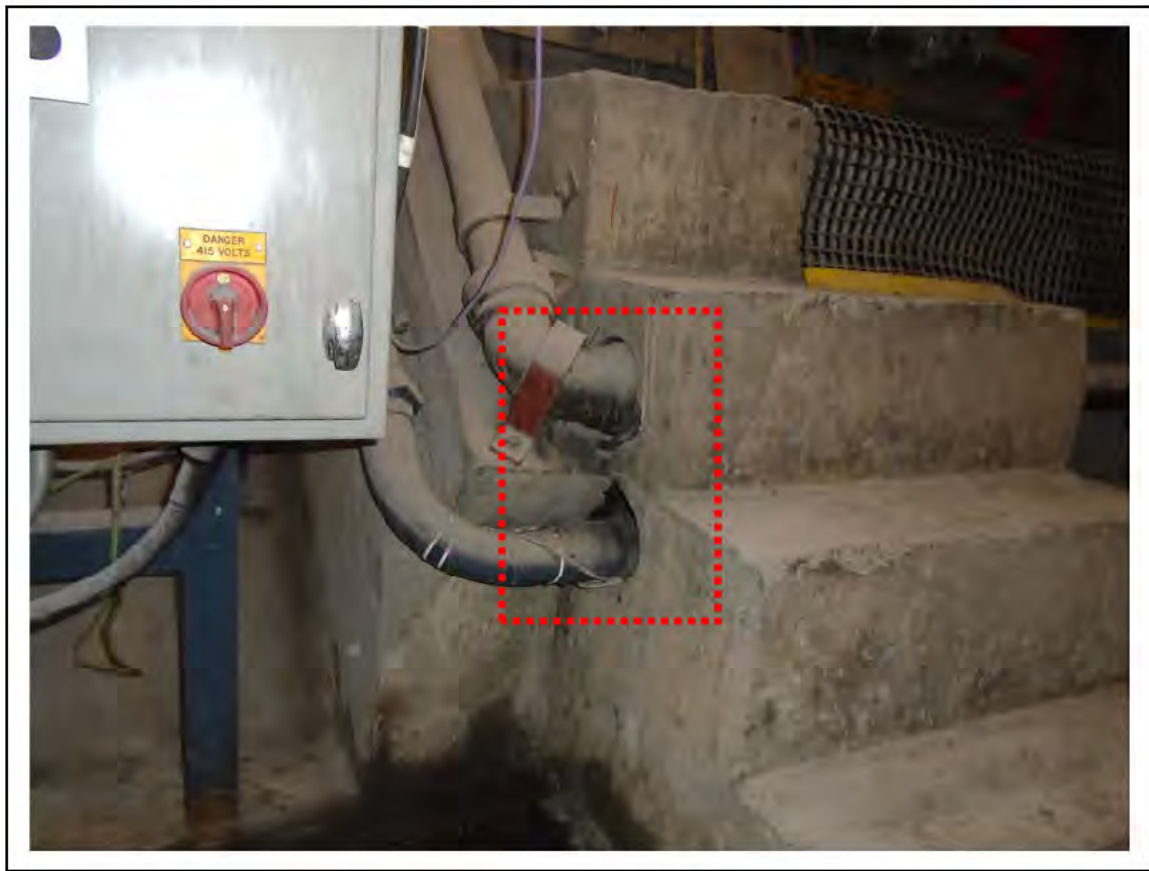
FIGURE 21: CONFIRMED ASBESTOS IN BITUMEN DUCTS IN LMC 6, 7, 8, 4/162 - DESCRIPTION & RESULT OF ASSESSMENT (SAMPLE REF. 100674/241110/17)
